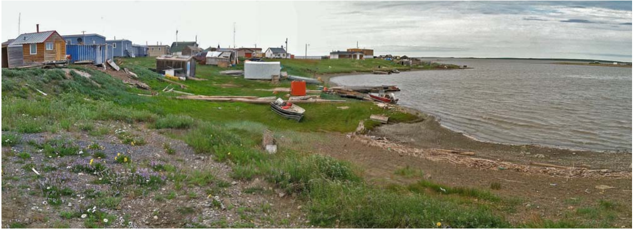
Shoreline buildings Tuktoyaktuk, NT
